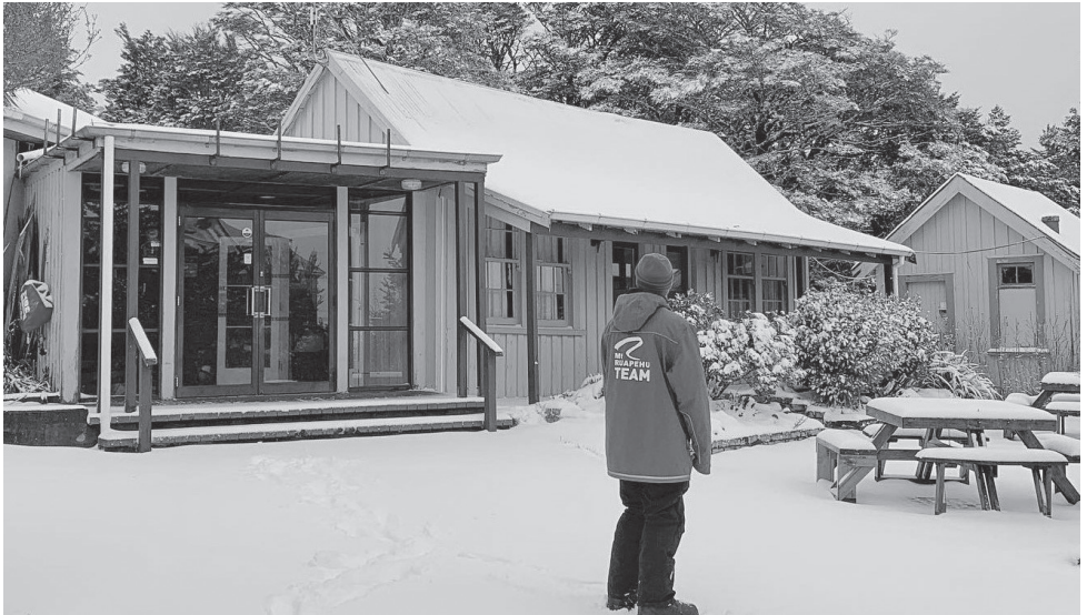
This café near The Chateau, seen in snow this season, has buildings which are close to 100 years old. The centre building was erected in 1925 as bunkrooms and is named Fergusson's Cottage after the Governor-General's wife Lady Alice Fergusson who stayed there. The building on the right is the original 1925 laundry, while the entrance to the left incorporates the original ablution block. Photo: RAL
