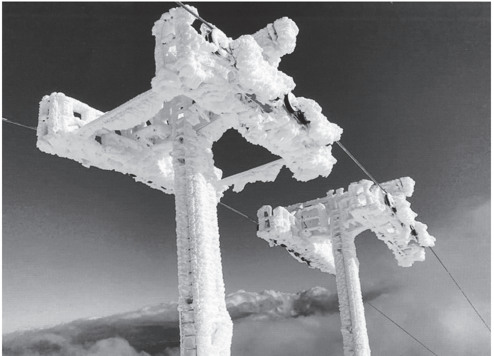
Upper: Stringing the wire on the Far West T-bar at Whakapapa. Lower: Ruapehu chairlift ice is the heaviest found at any skifield worldwide. Photos: RAL.
